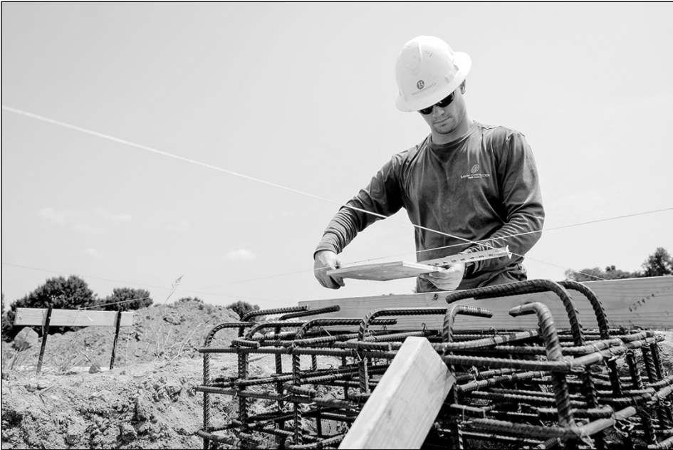
UT Martin rising senior Seth Edwards is shown taking a measurement to align the base plate pattern in the pier. Edwards said he is considering a career as a construction project manager.
