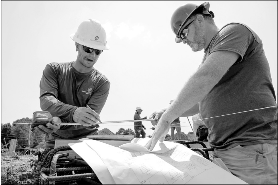
UT Martin rising senior Seth Edwards is shown at the TEST Hub construction site, working with his project manager, JT Donovan, as they go over base plate patterns to set piers.
