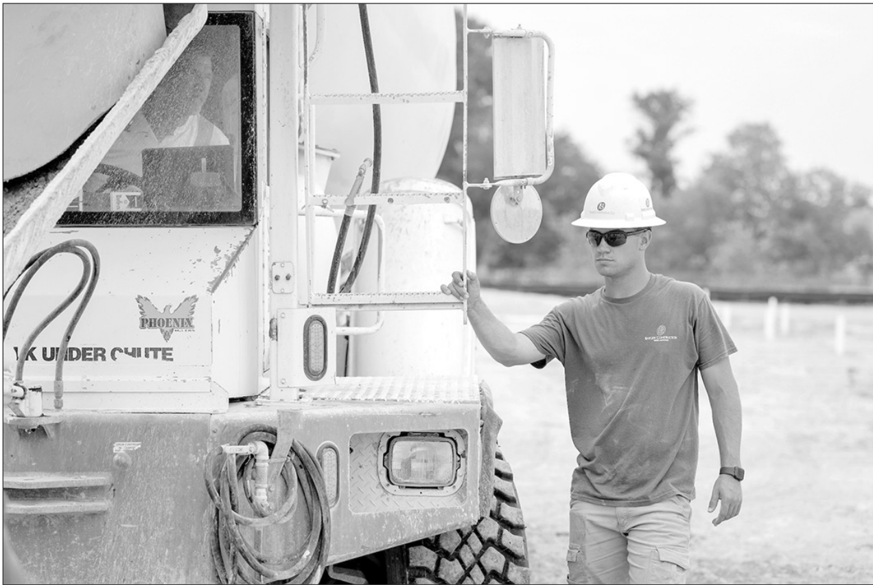
UT Martin rising senior Seth Edwards directs the concrete truck operator where to move the chute to pour concrete while working the TEST Hub site at UT Martin.
